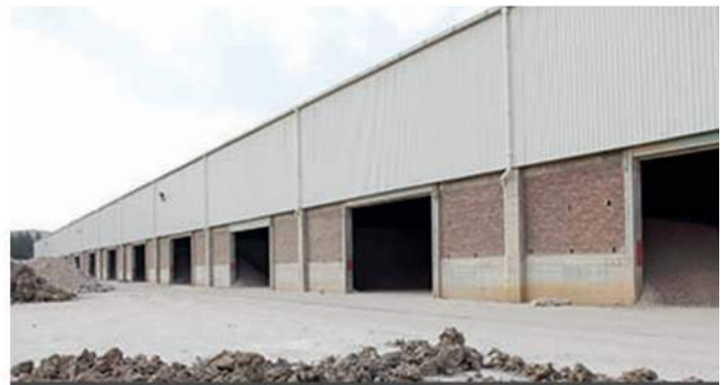
The semi-product indoor repository with storage capacity of 150,00 tons.
