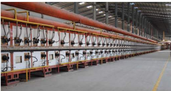
Domestic longest roller klin (260 meter) with 428 firing units
